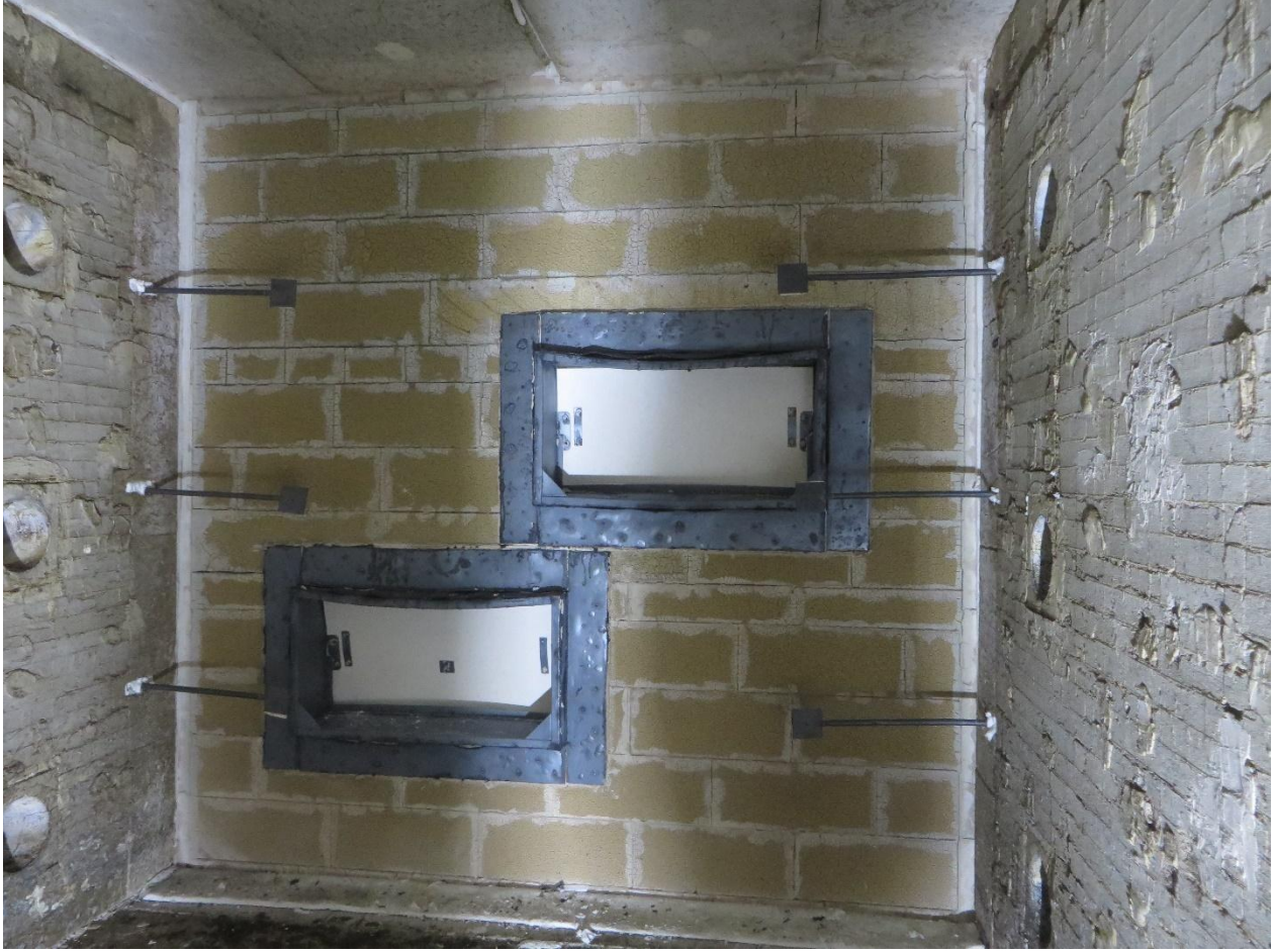
Photo C4: Exposed side after the fire test
